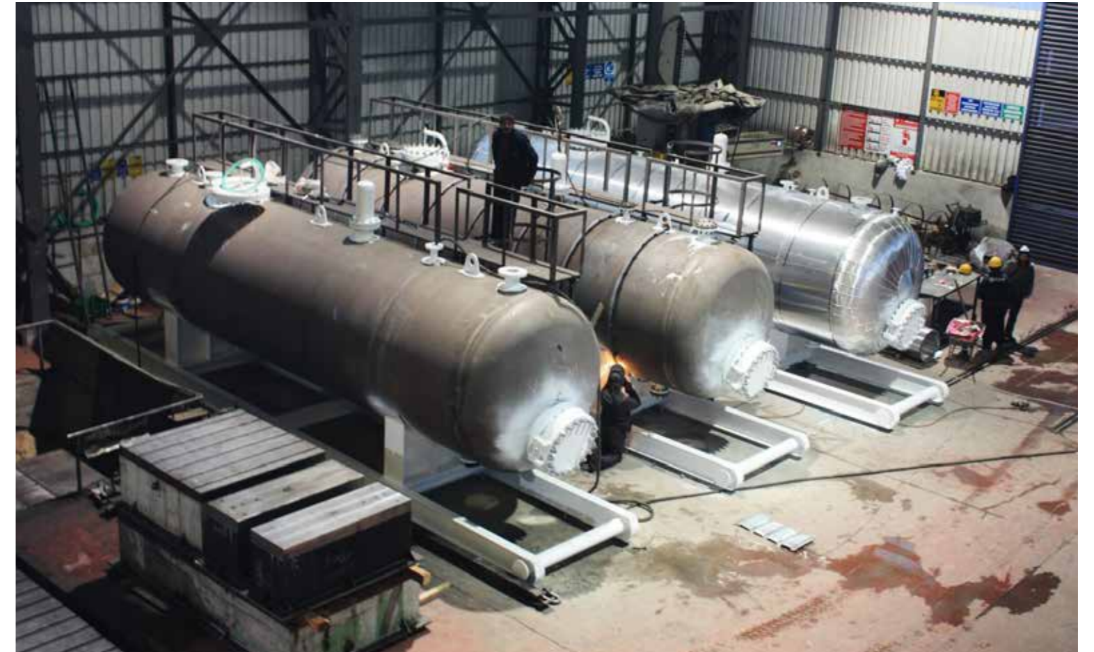
TPAO Adiyaman & Batman, Turkiye Contractor: ALSTOM Hydro
