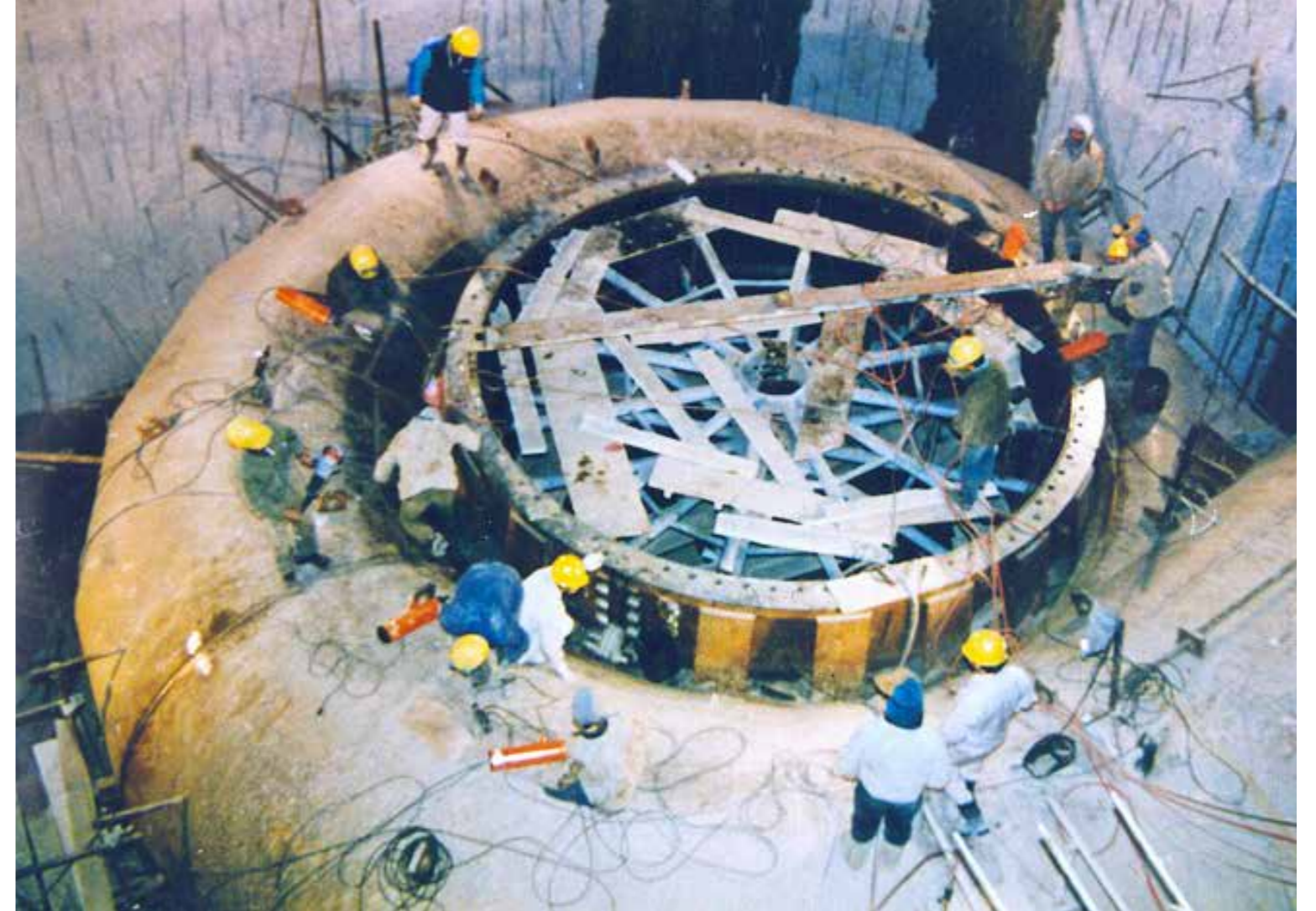
Sır DAM and HEPP, Turkiye (283 MW) Contractor: TOSHIBA Co.
