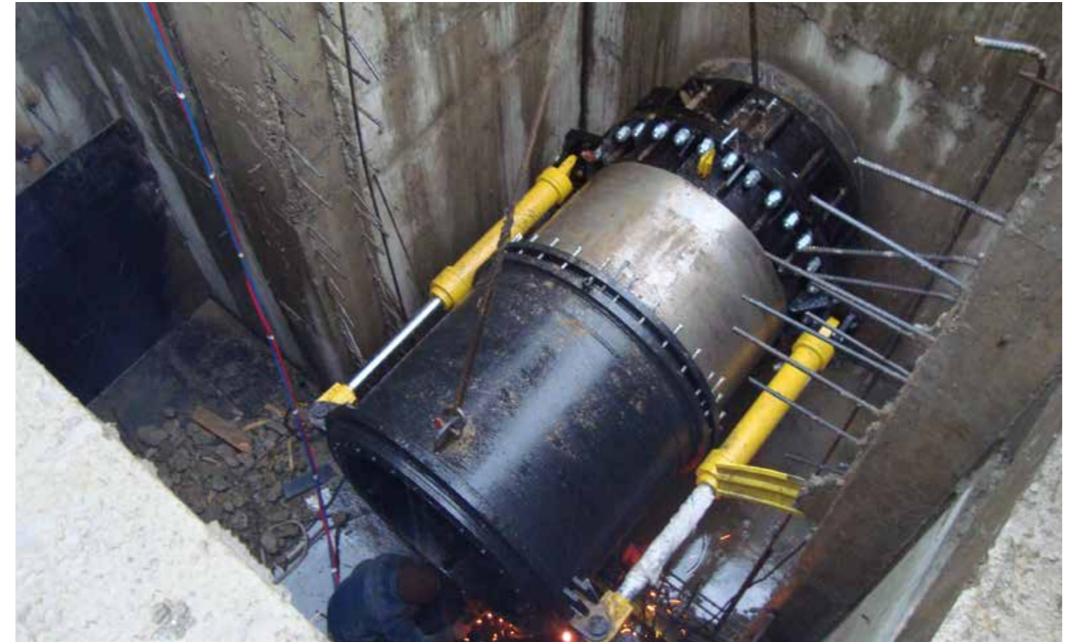
Aksu HEPP, Turkiye Contractor: KALYON CONSTRUCTION
