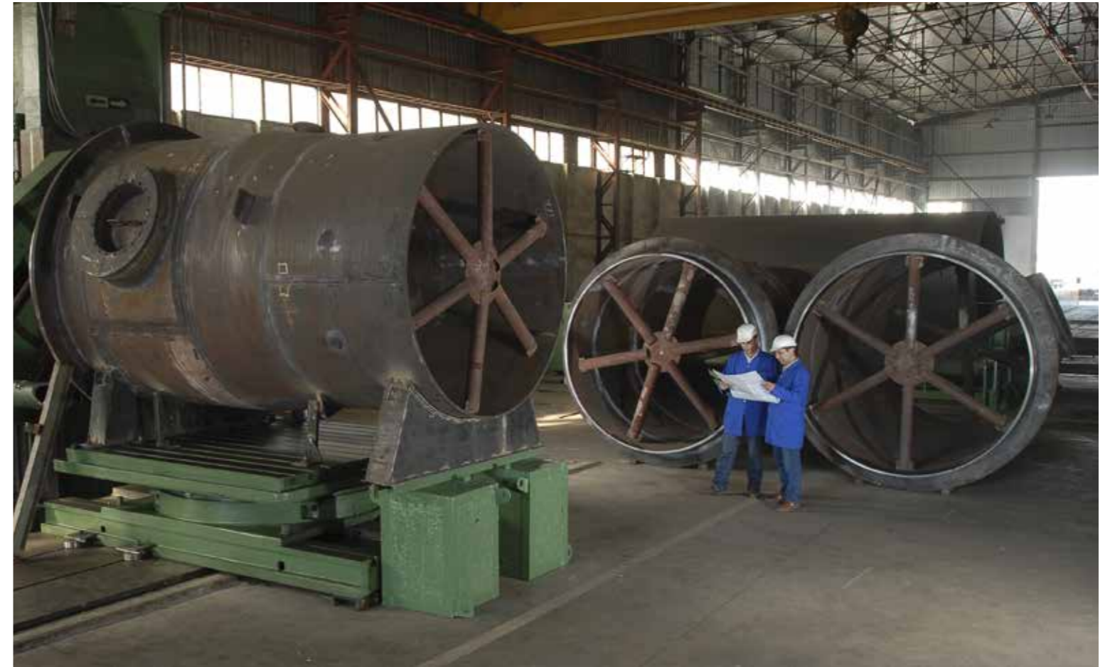
Akköy HEPP, Türkiye (2 x 116 MW) Contractor: VOITH Hydro
